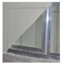
Installation example The door is attached to the aluminum profile with screws and stitched on the front plasterboard.
